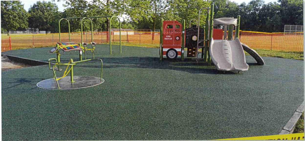
Entire Playground System Minus Swings and Completed Poured in Place Safety Surface
