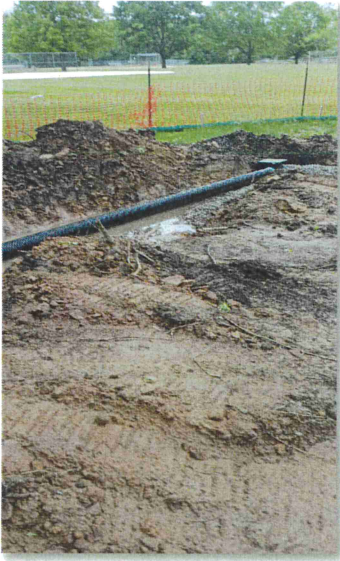
Pipe Insall at Existing Drain
