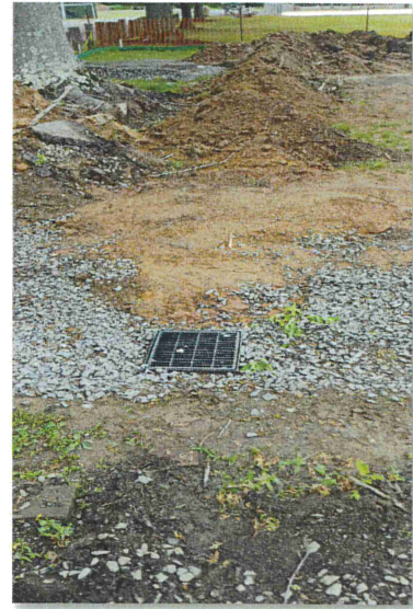
Example of Inlet at Grade
