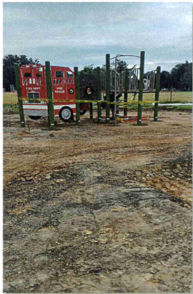
Initial Structure Insallation
